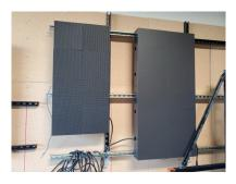
Struts will be mounted using 3/8 Bolts and 3/8 struts wing nuts , then cabinets will be secured to one another using 3/8" nuts and bolts
