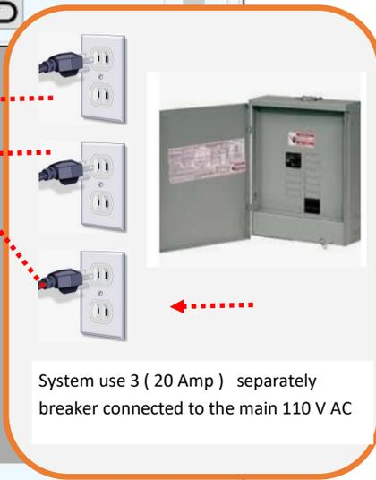
System use 3 ( 20 Amp ) separately breaker connected to the main 110 V AC
