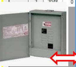
System use 5 ( 20 Amp ) separately breaker connected to the main 110 V AC source
